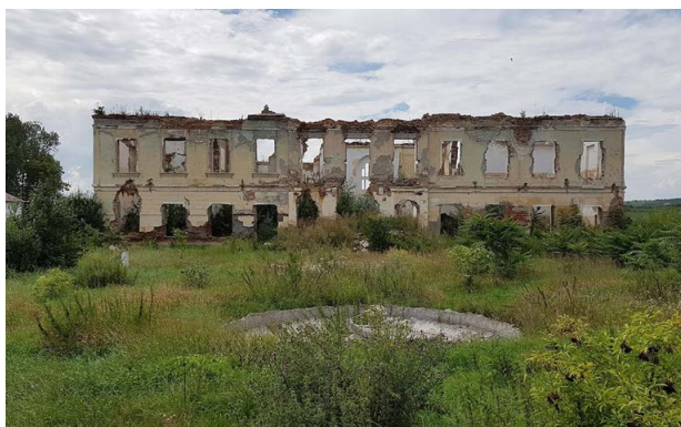
FIGURE 2 The ruins of Huszár castle and its gardens, in Apalina, Mureș county
