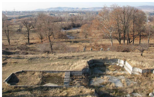
FIGURE 3 The park of the Cantacuzino Palace in Florești, Prahova County, prior to the development of a preservation strategy in 2018
